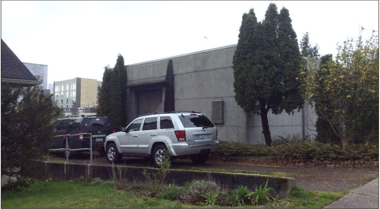
Photo 6 – Avalon Substation, East Elevation. View to the southwest. (Source: City Light Collection, 2016)
