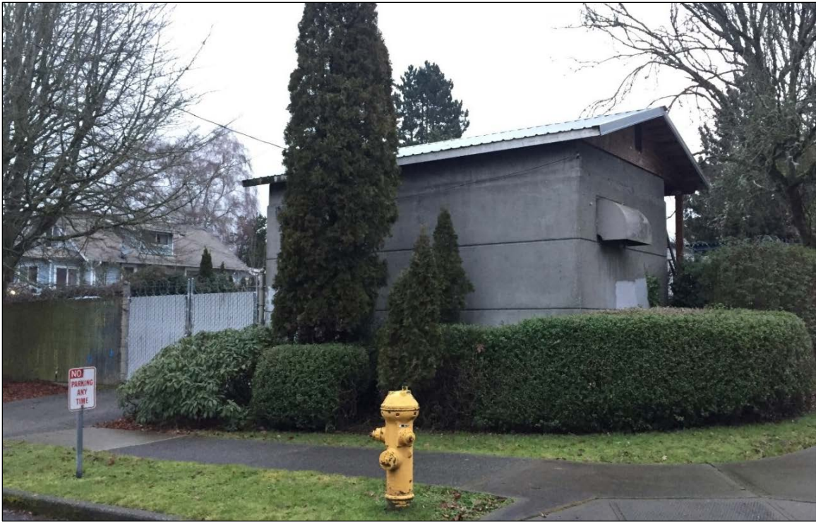
Photo 24 – Roxbury Substation, West Elevation. View to the northeast. (Source: City Light Collection, January 26, 2017.)
