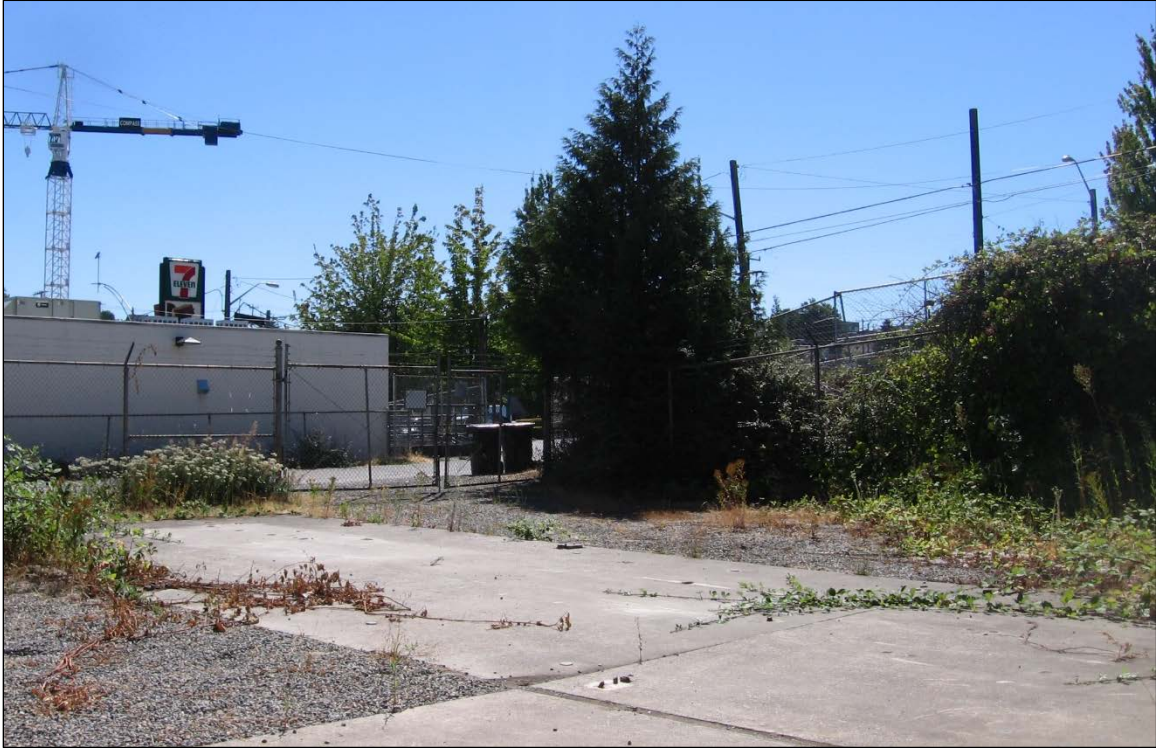
Photo 8 – Avalon Substation, South Yard Area. View to the southwest toward 35 th Avenue SW. (Source: City Light Collection, 2016)
