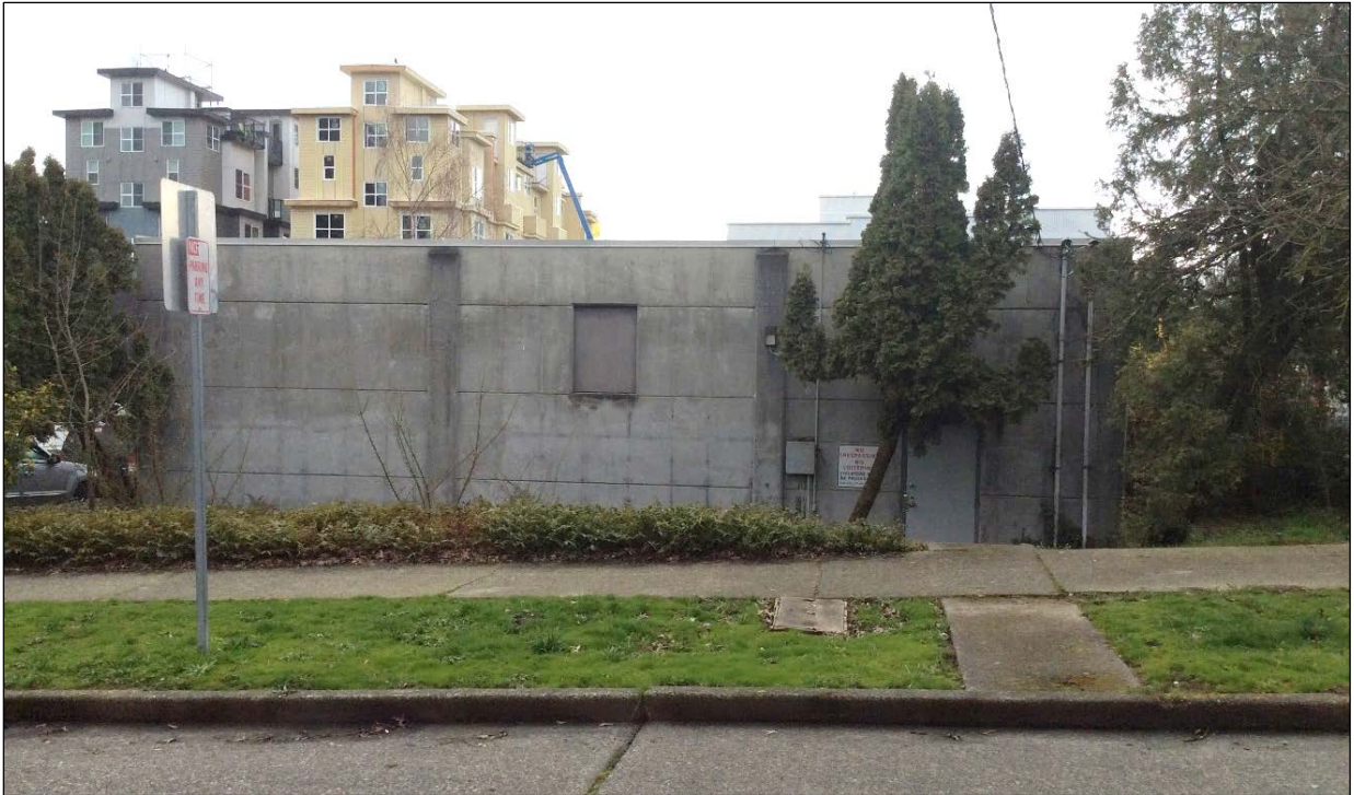
Photo 5 – Avalon Substation, North Elevation. View to the south. (Source: City Light Collection, 2016)
