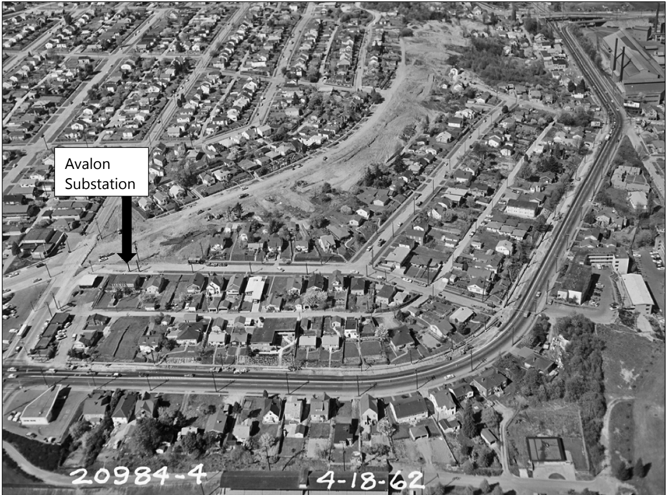
Figure 16 – Aerial View SW Spokane St. Interchange, April 18, 1962. (Source: SMA #71143)
