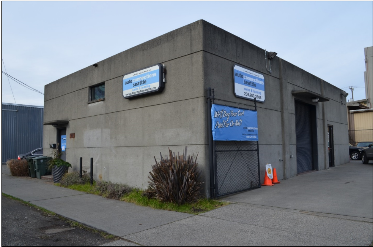
Photo 16 – Leary Substation, Southeast Elevation. View to the northwest. (Source: City Light Collection, January 13, 2017).
