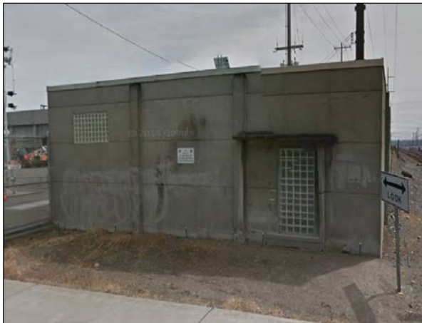
Photo 29 – South Rectifier, North Elevation in 2014. (Source: Google street view, June 2014.)
