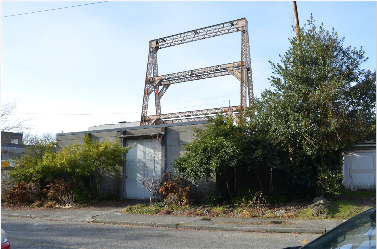
Photo 19 – North Substation, East Elevation. (View to the southwest. (Source: City Light Collection, January 13, 2017).
