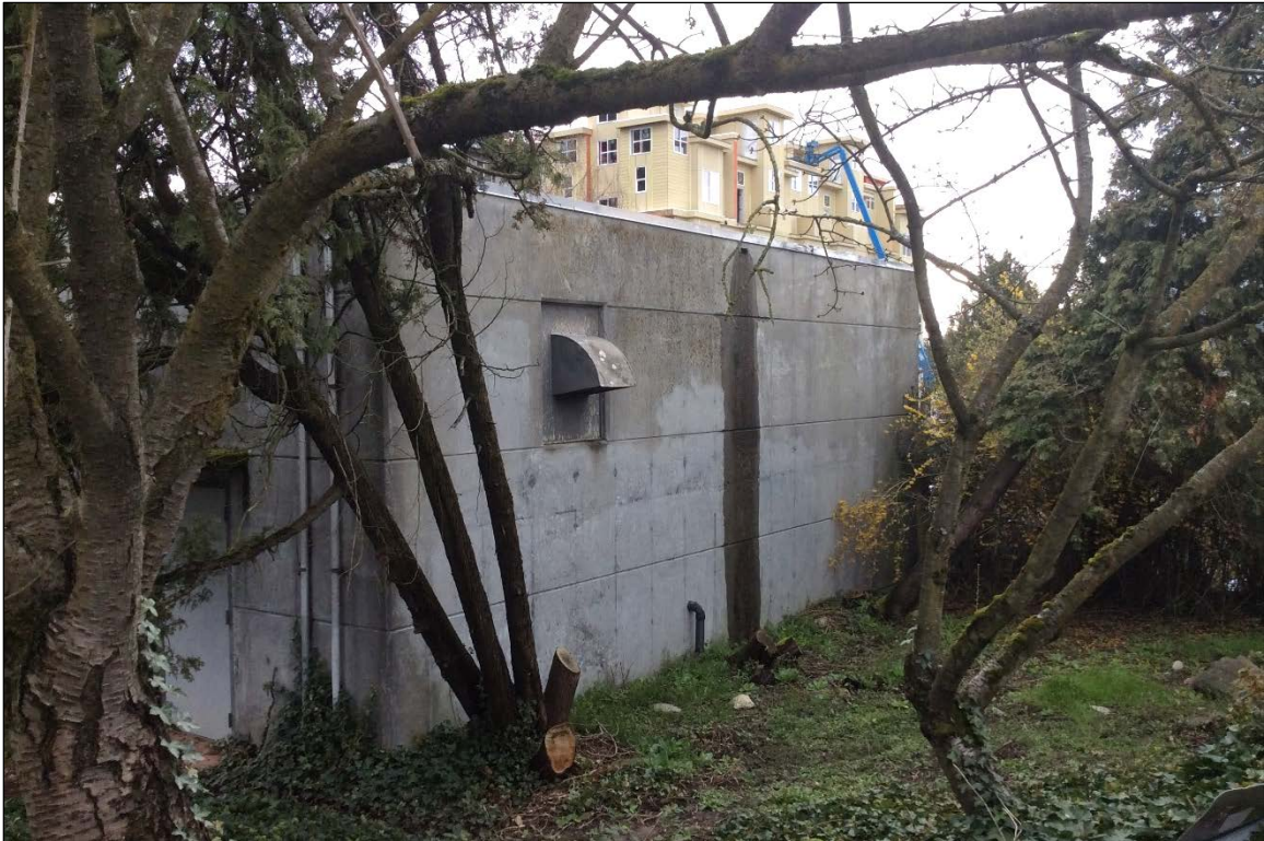
Photo 9 – Avalon Substation, West Elevation. View to the southeast. (Source: City Light Collection, 2016)
