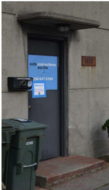
Photo 17 – Leary Substation, South (Main) Entry
