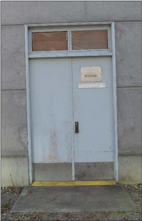
Photo 34 – University Rectifier 1941 Entry Door.
