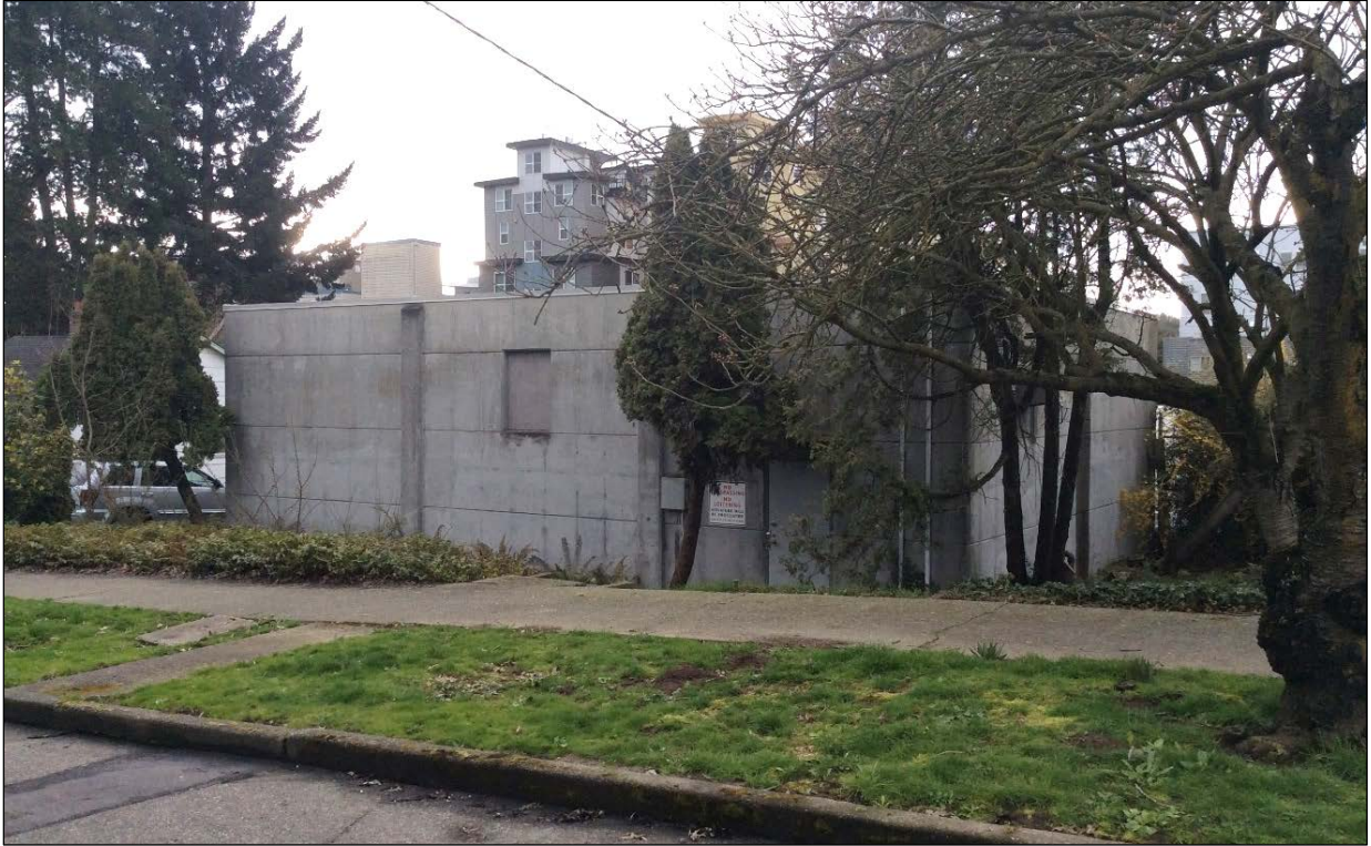
Photo 4 – Avalon Substation, Northwest Elevation. View to the southeast (Source: City Light Collection, 2016).
