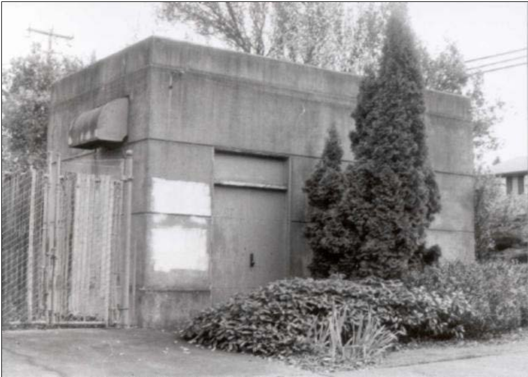
Photo 26 – Roxbury Substation in 2000 (Source: DON Survey, 2000.)
