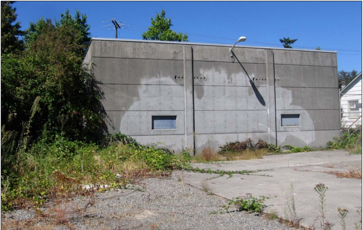
Photo 7 – Avalon Substation, South Elevation. View to the north. (Source: City Light Collection, 2015)
