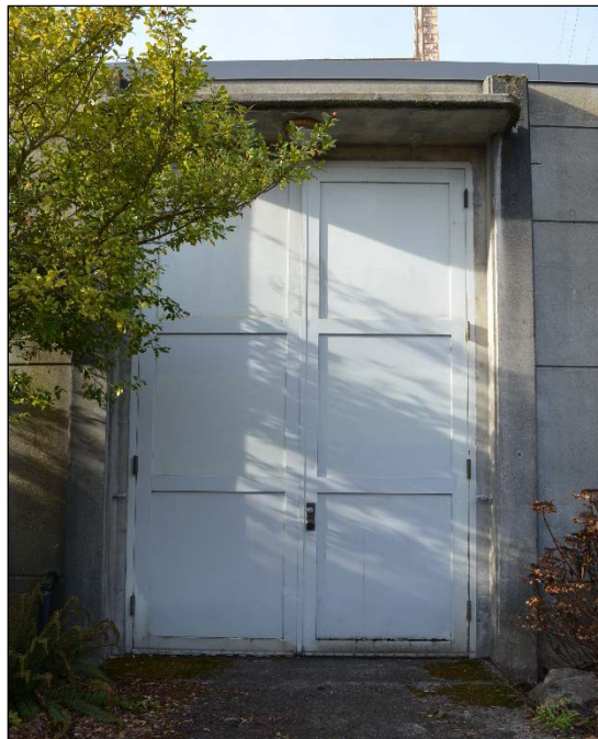
Photo 20 – North Substation, East Entry Porch and Double Door Details (Source: City Light Collection, January 13, 2017).
