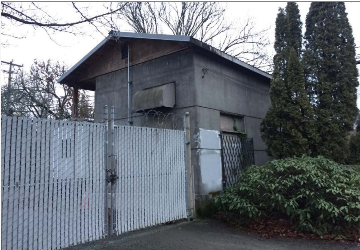
Photo 25 – Roxbury Substation, Northwest Elevation. View to the southeast. (City Light Collection, January 26, 2017.)
