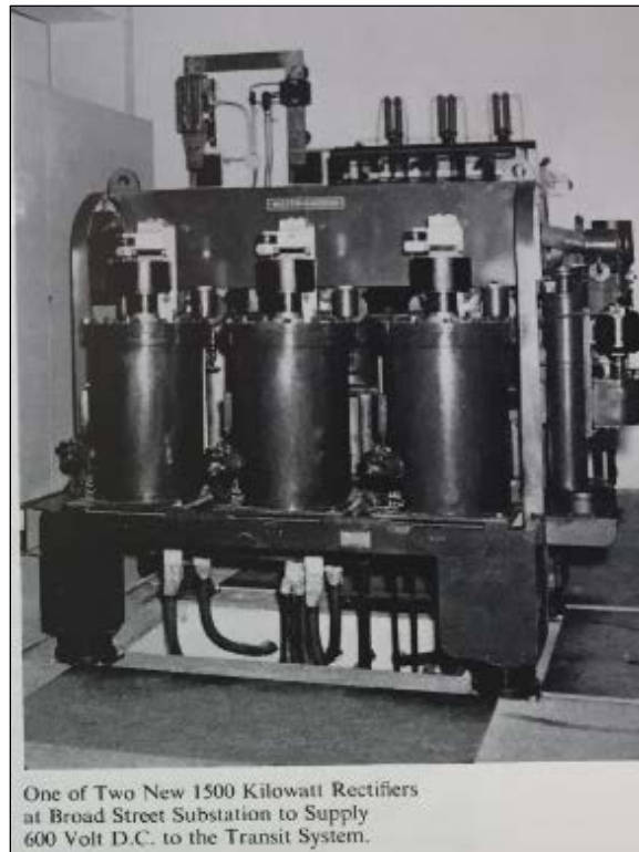
Figure 5c – One of Two City Light’s New Rectifiers at Broad Street Substation (Source: City of Seattle, Department of Lighting, Annual Report for the Year Ended December 31, 1951, 13.)
