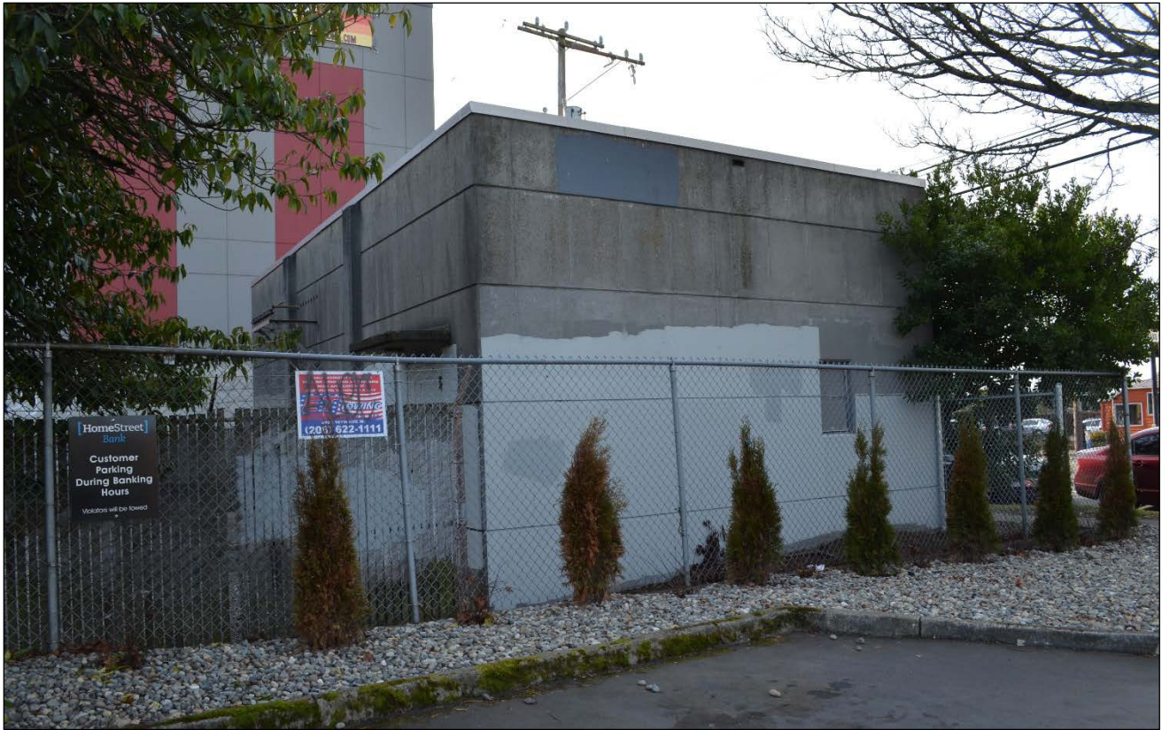
Photo 21 – Olympic Substation, Northeast Elevation. View to the southwest. (Source: City Light Collection, January 13, 2017).
