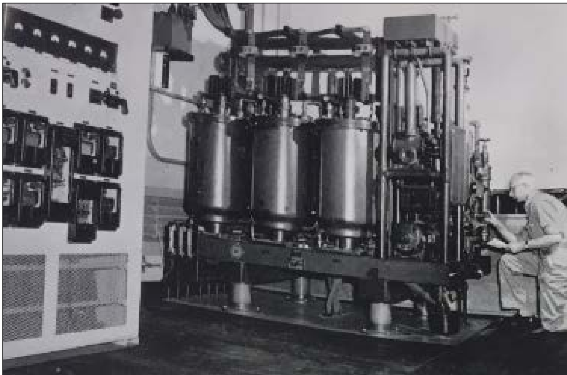
Figure 5d – University Rectifier’s 1,000 kW Mercury-Arc Unit (Source: City of Seattle, Department of Lighting, Annual Report for the Year Ended December 31, 1954, p.16.)
