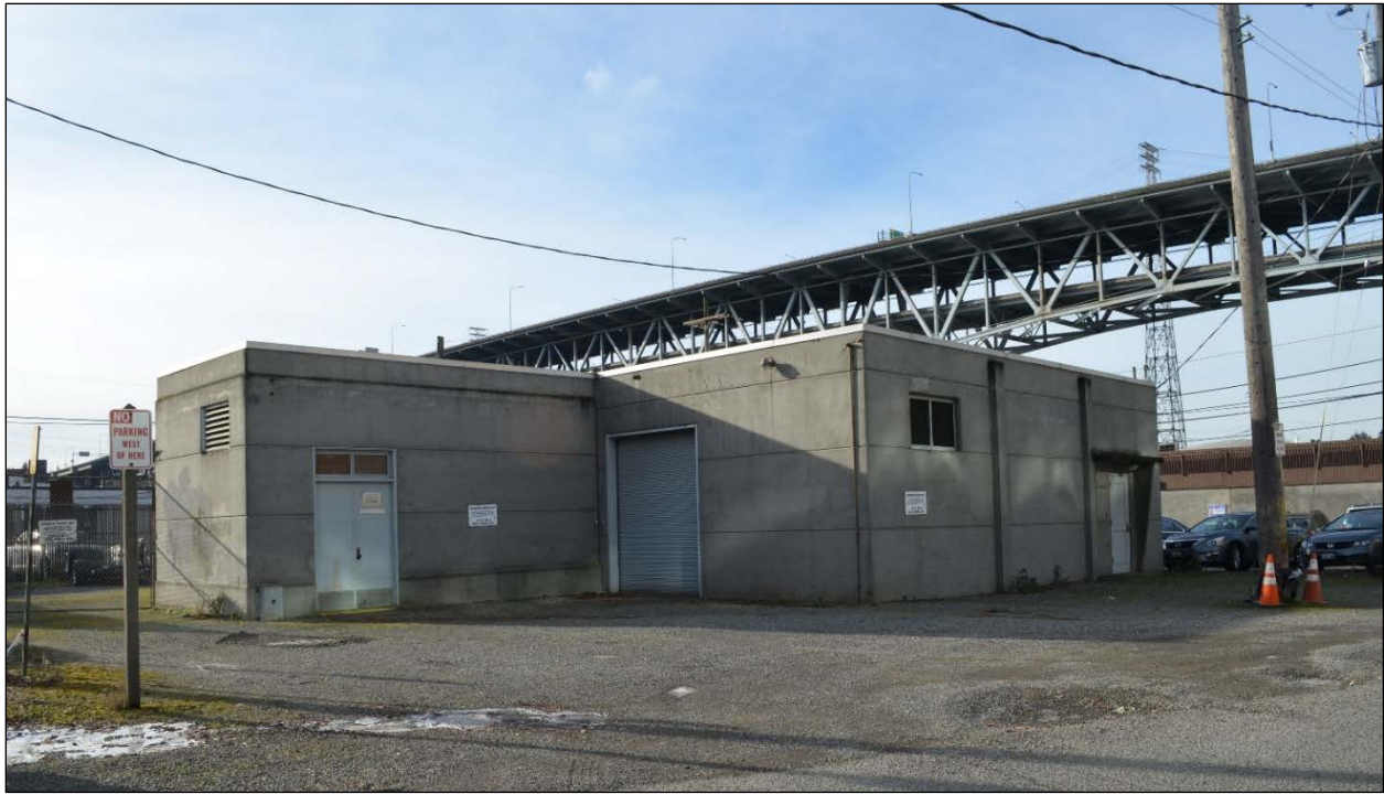
Photo 31 – University Rectifier, Northeast Elevation View to the southwest. Smaller building on the left was built in 1941, larger on the right in 1952. (Source: City Light Collection, January 13, 2017).
